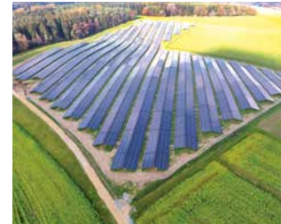
› Ground-mounted system Sillaching approx. 111 MWp
