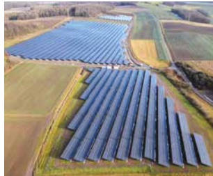
› Ground-mounted system Theinfeld approx. 112 MWp
