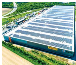
› Rooftop system Dieburg approx. 16 MWp
