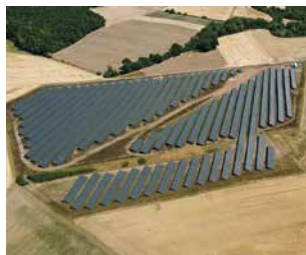
› Ground-mounted system with storage, Reckertshausen approx. 110 MWp
